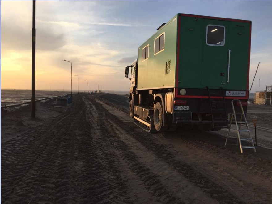
Zelazny Most Tailings Dam (Poland) November 2019
