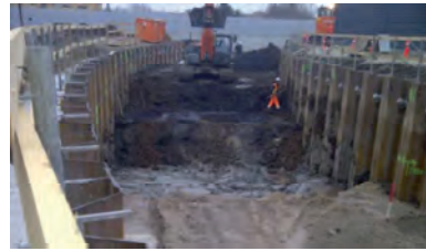
Figure 11. Excavation of organic soil [3]
