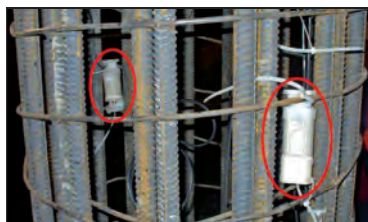
Figure 4. MDS installation in the body of a cast-in-place pile
