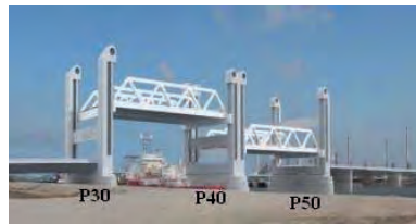
Figure 1. Artist impression new Botlek lifting bridge with main piers P30, P40 and P50. Source: Quist Wintermans Architecten
