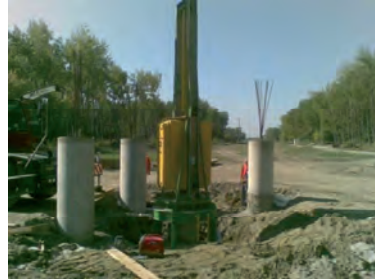
Figure 8 Dynamic pile load testing on the test field P2
