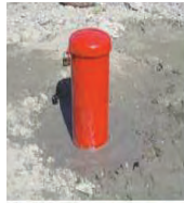
Figure 5. Photo of cone protection of inclinometer tube
