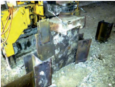
Figure 7. Hammering of plate in King Post Wall under bridge [3].
