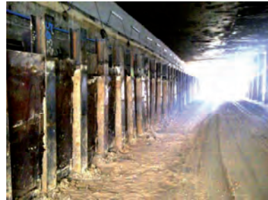
Figure 9. King post wall under bridge after excavation [3]
