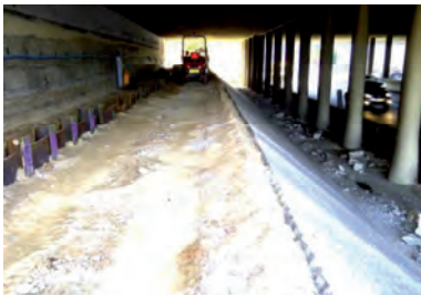
Figure 8. King post wall under bridge before excavation [3].
