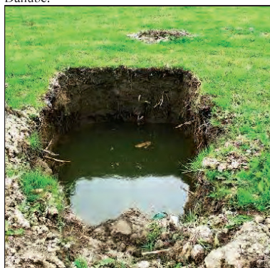
Figure 2. Existing excavation pit.
