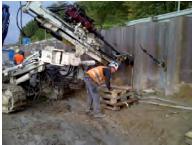
Figure 10. Boring of ground anchor [3]
