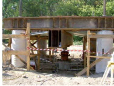
Figure 2 Apparatus for static pile load testing.
