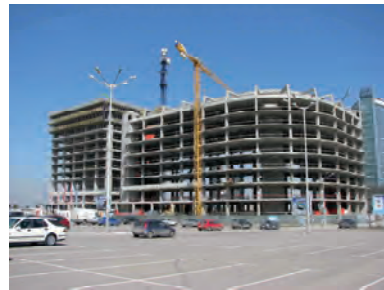
Figure 10. Construction progress at the middle of May 2012
