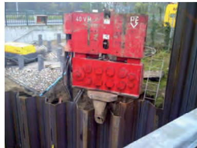
Figure 6. Vibrating from crane [3].
