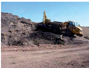
Figure 2. Coal being extracted from a seam exposed in an earthworks cut.
