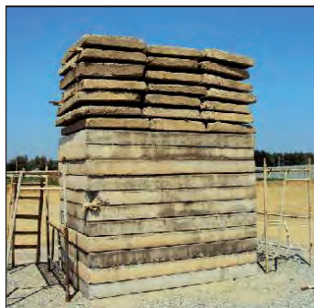
Figure 6. Loading with concrete slabs.
