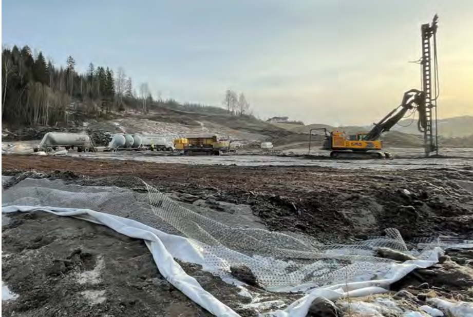
Figure 7 Soilmixing performed by SMG. Credit T. Bjørhusdal.
