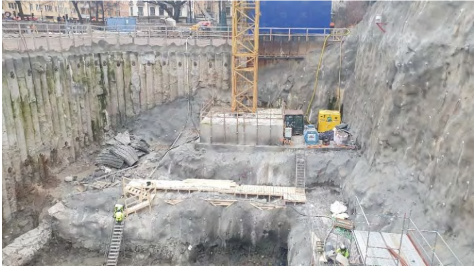
Figure 81 Secant pile wall, facing south and west, rock slope facing north.
