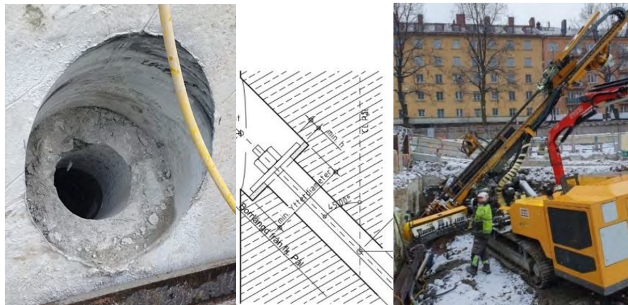
Figure 77 Left and middle– holing in each secondary pile for further anchoring. Right- ongoing drilling for anchoring.
