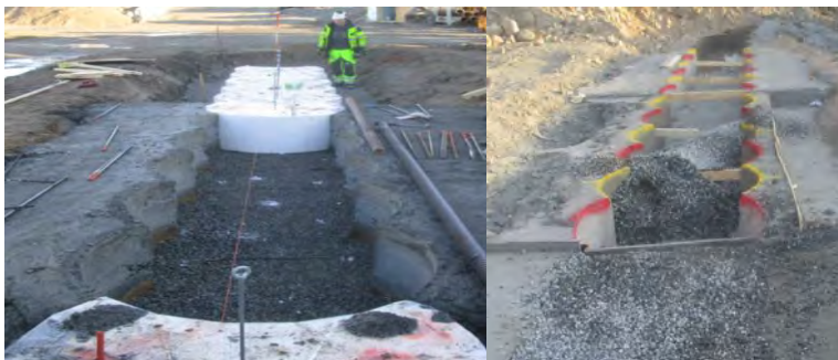
Figure 75 Pictures showing a typical drilling template for aiding alignment.
