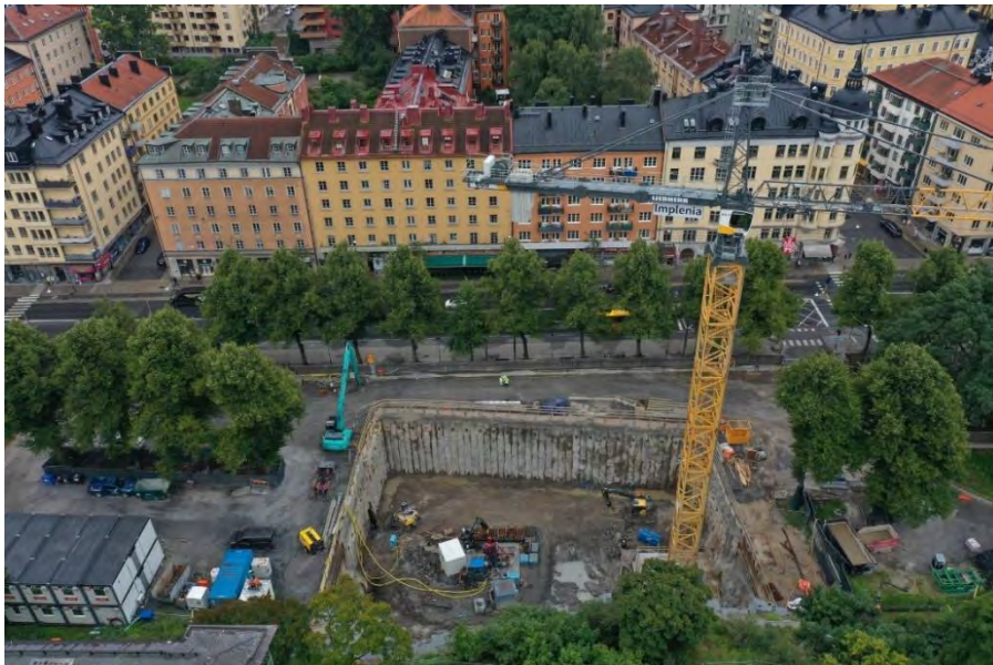
Figure 71 Picture showing time for installation of anchor level 2 as well as ongoing raise boring for the elevator shaft.
