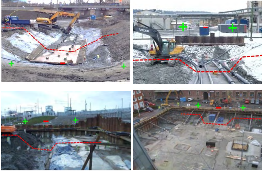
Figure 1. Some typical situations where 3D-effects have been incorporated in design in order to achieve satisfying stability conditions in temporary excavations. Upper left: A battered excavation with a limited horizontal extent. Upper right: A cantilever sheet pile wall next to trafficked railway tracks. Lower left: A cantilever sheet pile wall supporting an excavation that progresses sequentially from right to left while simultaneously casting a concrete slab. Lower right: A sheet pile wall supported by struts while excavating and casting a concrete slab sequentially.
