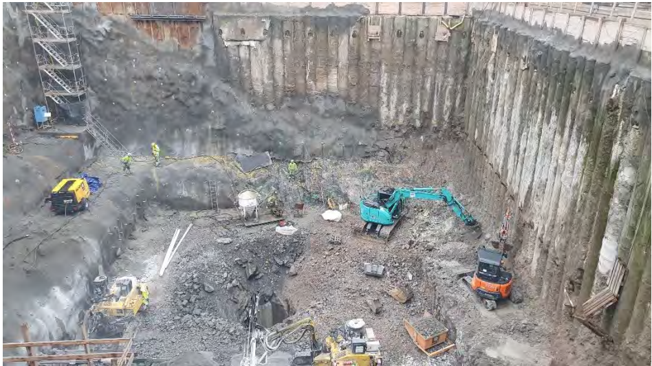
Figure 80 Secant pile wall, facing east and south.
