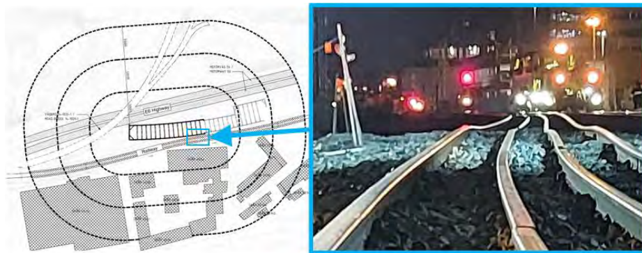
Figure 24: Risk zone of 50 m, 100 m and 150 m distance from the location of groundwork execution. During installation of jet grouting heave may appear fast and with significant impact.
