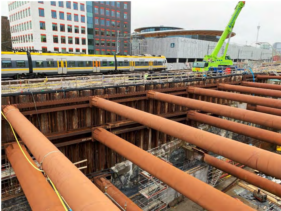
Figure 21: Live railway next to the strut supported deep excavation for the Västlänken-tunnel.
