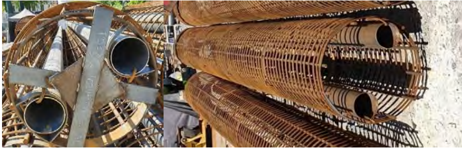
Figure 74 Pictures showing reinforcement cages incl. steel casing for curtain grouting.
